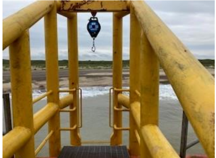
Push on CTV ladder system (right – inertia reel and grating in place at top of ladder)
