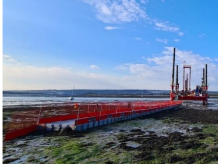
Plastic jet float walkway in use across shallow/dried out area.
