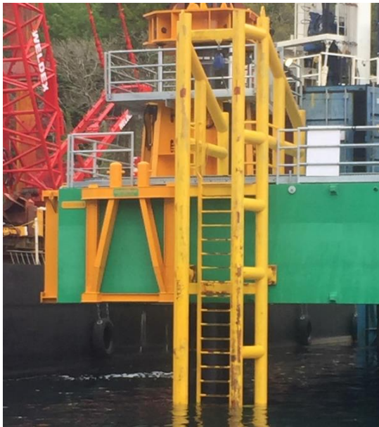
Push on CTV ladder system (right – inertia reel and grating in place at top of ladder)
