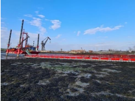
Plastic jet float walkway in use across shallow/dried out area.
